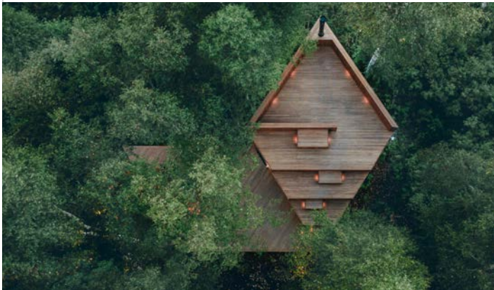
Unoiled Thermory Benchmark thermo-ash decking after installation
