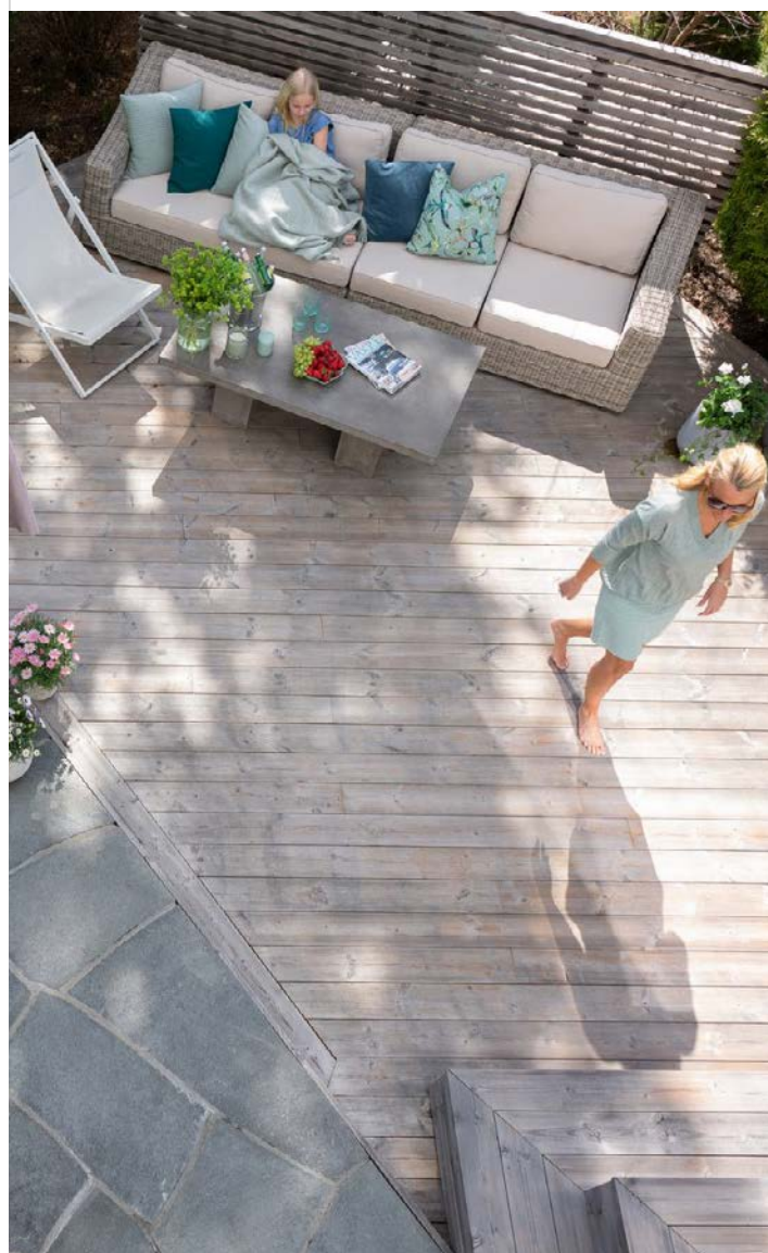
Unoiled Thermory Benchmark thermo-pine decking after 1 year Photo and distribution: Moelven Norway
