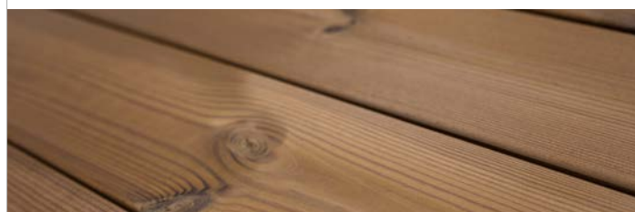
Unoiled Thermory Benchmark thermo-pine decking after installation
